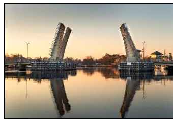
Medium Span Category Elizabeth City Bascule Bridge- Modjeski and Masters, Inc.
