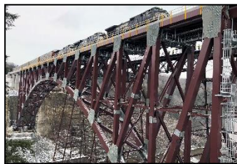
Long Span Category Portageville Railroad Bridge- Modjeski and Masters, Inc.
